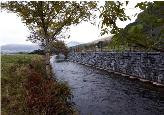
Completed downstream retaining wall
