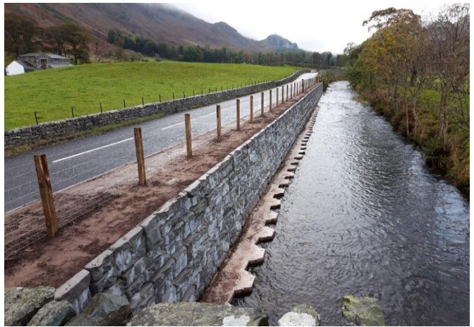
Completed upstream retaining wall
