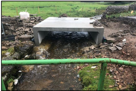
Installation of precast concrete units on riverbed
