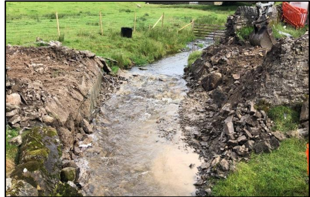
Removal of existing bridge
