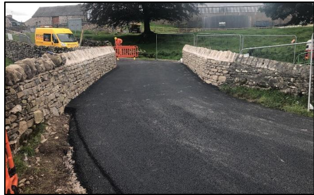
New carriageway constructed and parapets to new bridge
