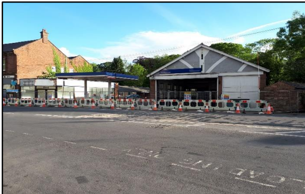
Site after soft strip prior to Demolition works.
