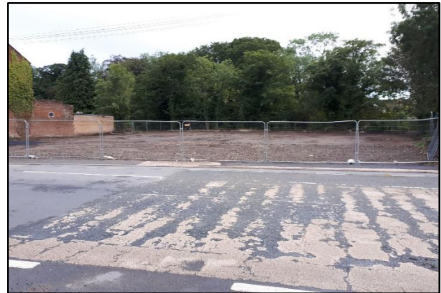
Completion of Demolition works and clearance from site
