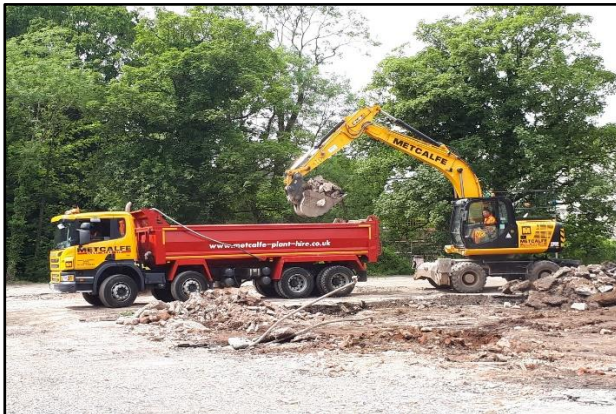
Removal of Demolition waste for recycling
