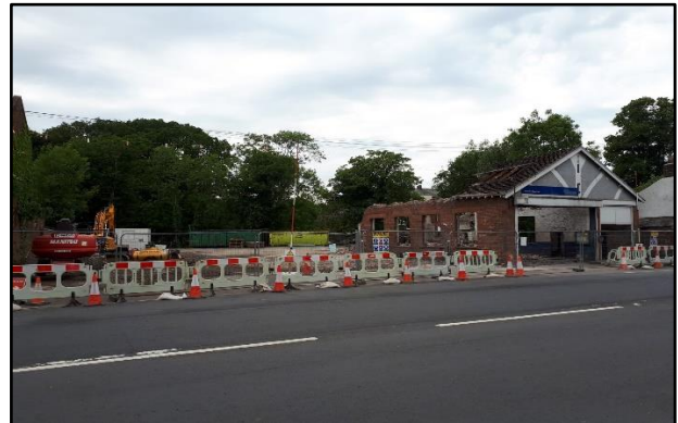
On-going Demolition works
